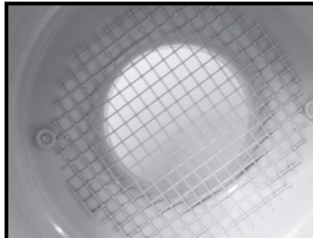
Step 8. Check inlet grille is clear.
