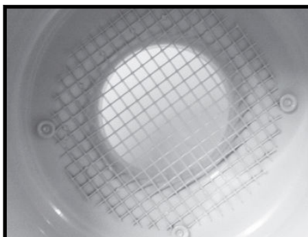
Step 17. Check inlet grille is clear.
